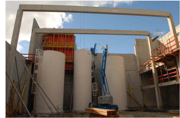
storage tanks, dec 2012
