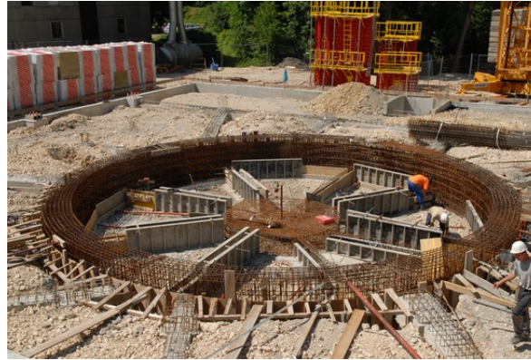
foundations platform: may 2012
