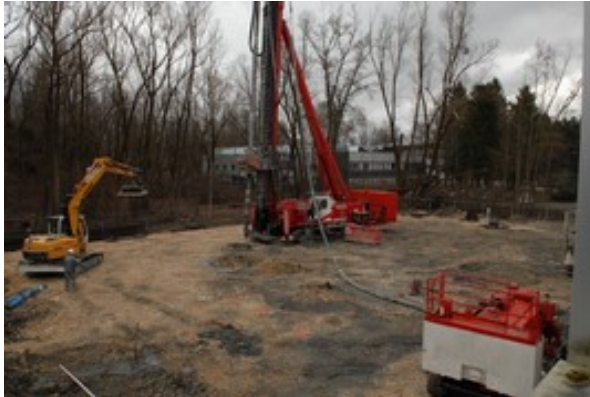
poles for foundations (20 m deep) feb. 2012
